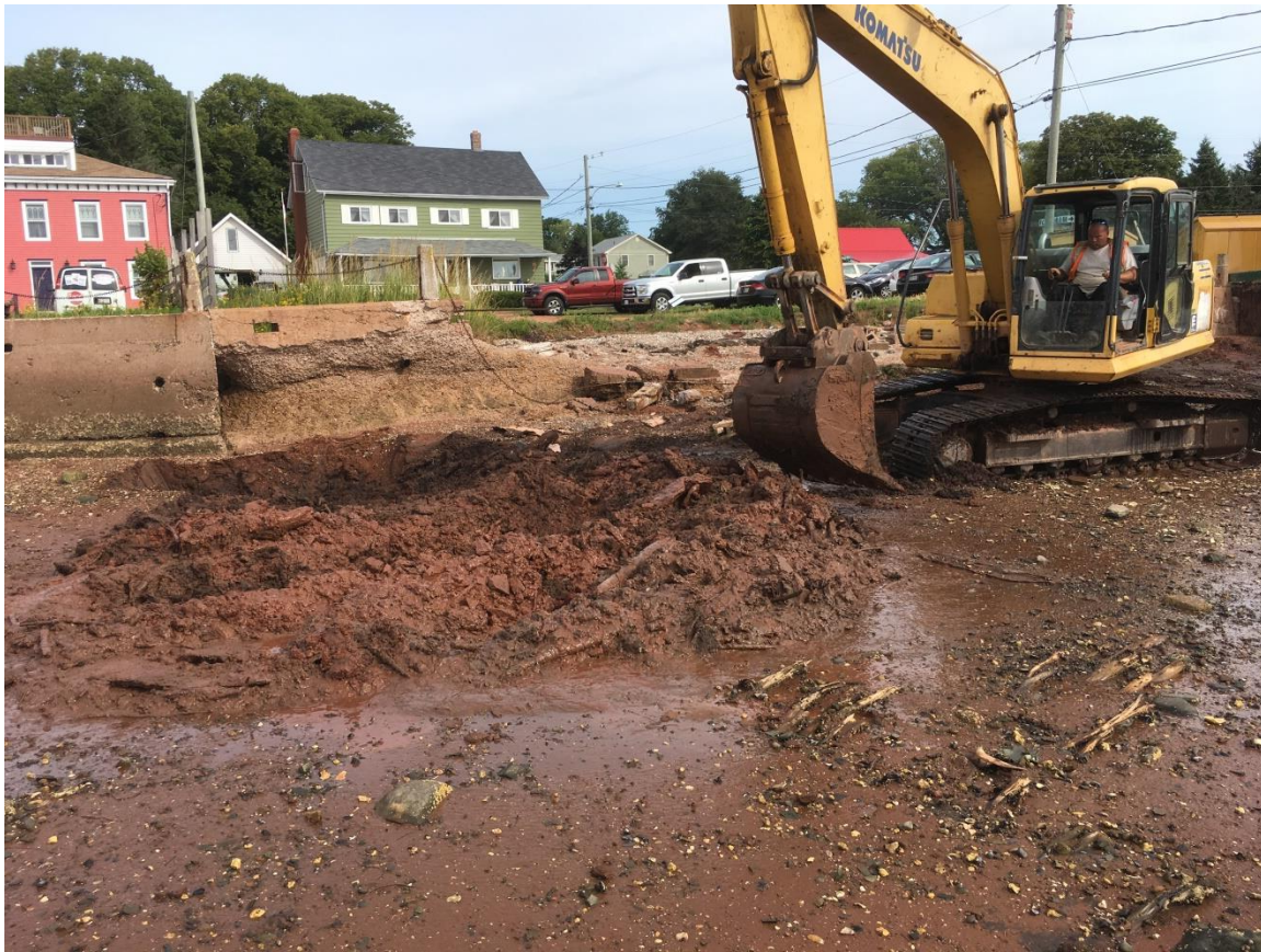
Figure 17 – Digging a test pit at the Community of Victoria seawall project site, August 30, 2017.
