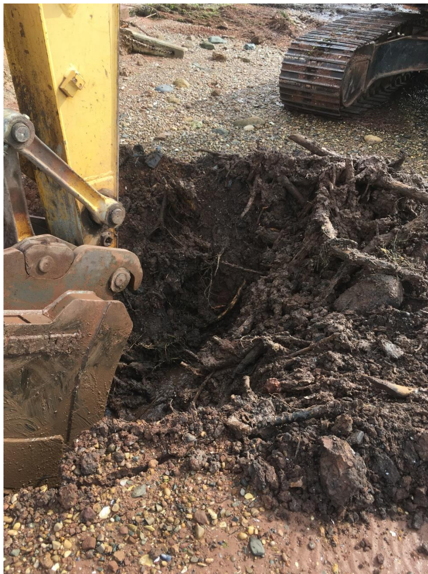
Figure 19 - Wood Debris from Old Wharf encountered in a test pit at the Community of Victoria proposed seawall site.
