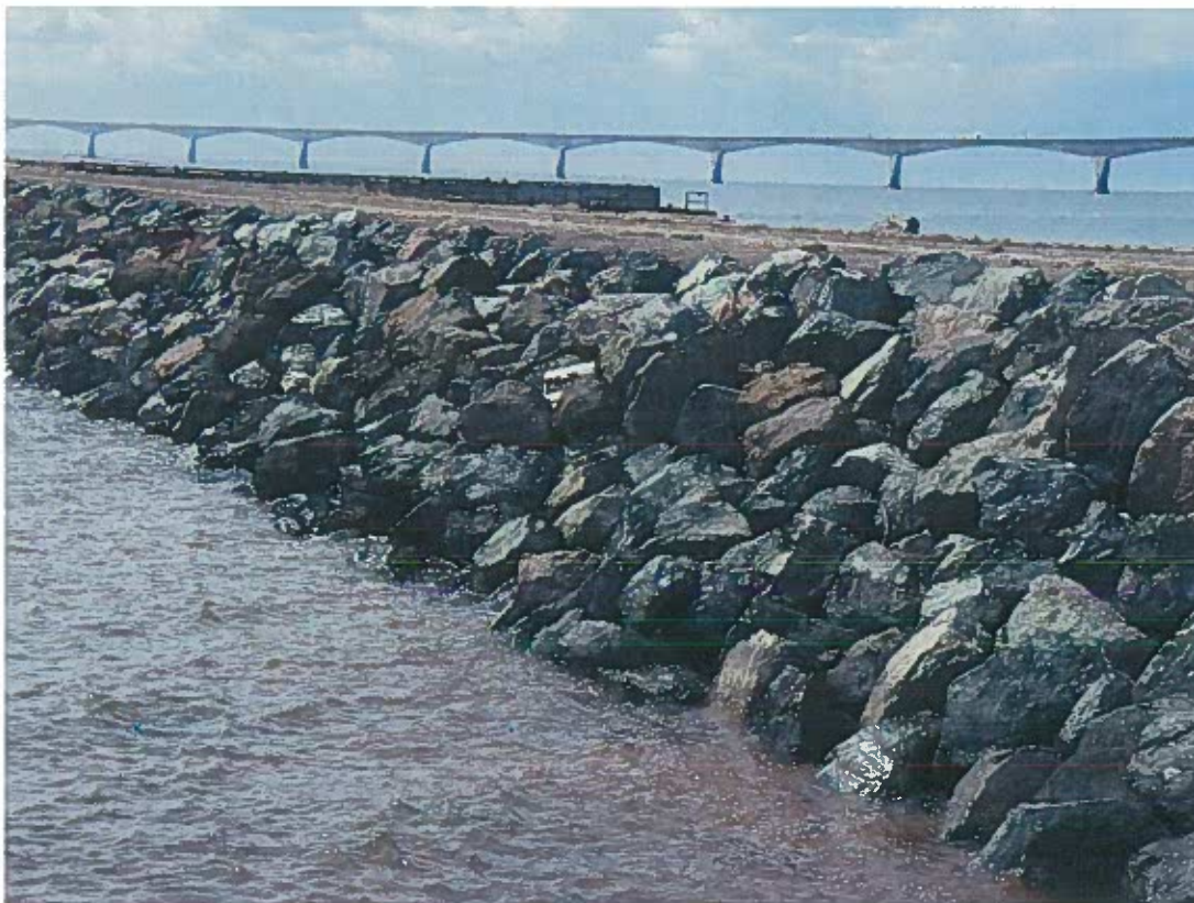
Rockfill portion of jetty
