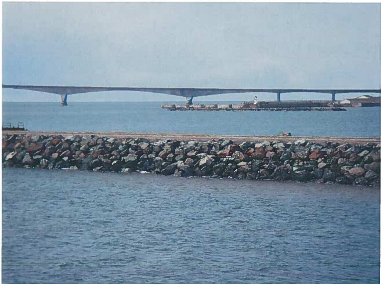
Rockfill portion of jetty with the Confederation Bridge in the background
