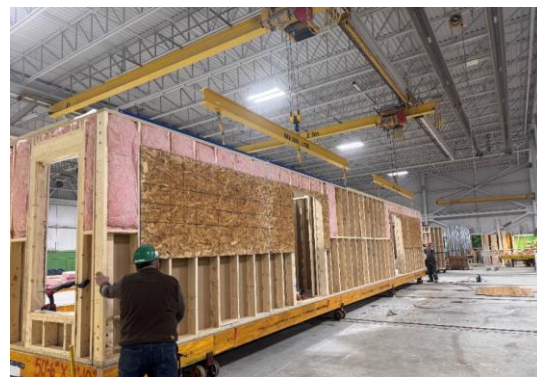
Modular unit in construction
