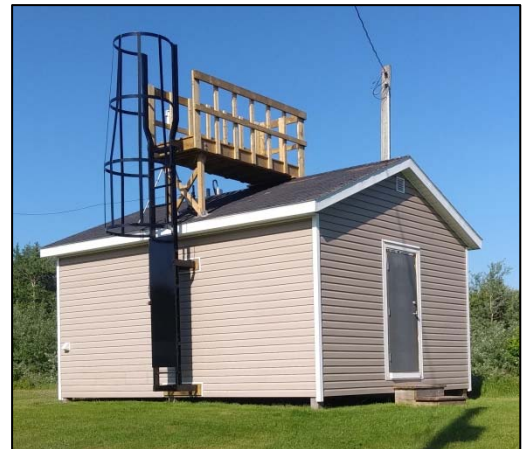
Figure 1 - PEI Air Quality Monitoring Station (Southampton)
