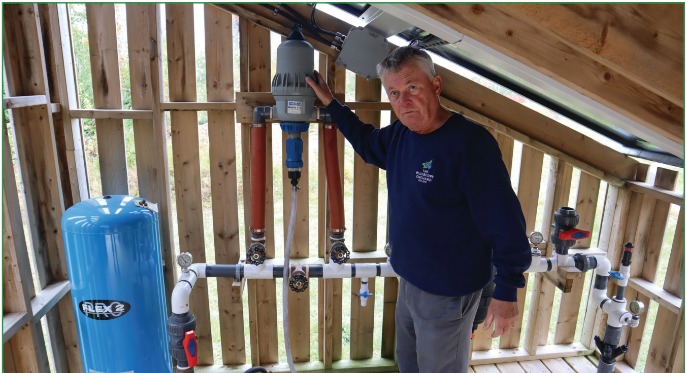
Gerard Morrison’s custom-built solar-powered irrigation and fertilization system has not only increased the volume and quality of his highbush blueberries, but also conserves water by directing it only where and when it is needed.
