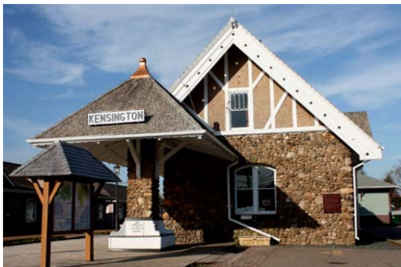
Kensington Railway Station Kensington
