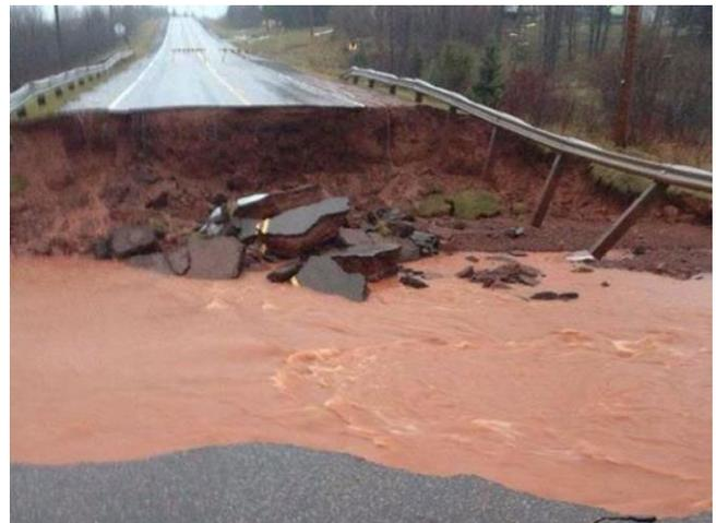
Figure 39. Road damage in West PEI after the December 2014 rainstorm [6].
