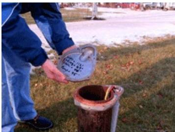
**STEP 3:** Inspect inside of well casing and cap for any signs of insect nests (earwigs, etc.) as they are a common source of coliform bacteria. If well is not sealed with a vermin proof cap, one should be installed.
