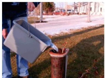
**STEP 5:** Pour the mixed chlorine solution into the well. If the well is buried with the old type of well seal cap, either expose the top of the well and remove the well cap pouring the solution directly into the well, or pour the solution through a clean funnel into the air vent or siphon through the vent (flush the air line with clean water after chlorination).
