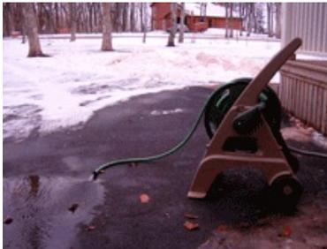
STEP 11: After time has passed, flush the system through an outside tap/hose until the chlorine odour has completely disappeared. Be careful not to discharge the chlorinated water in areas where it can harm vegetation (e.g. vegetable gardens). **DO NOT** discharge chlorinated water into the septic system.
