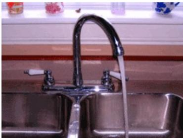
STEP 12: Allow the water to run through each household fixture individually until the chlorine odour is gone.
